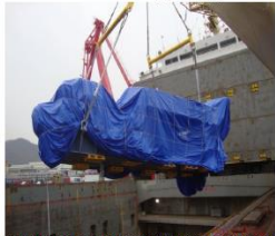
VIEW OF MAIN ENGINE UNDER LOADING IN NO. 2 LOWER HOLD.
